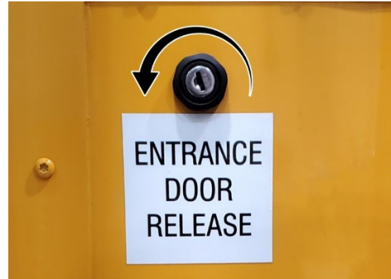
Figure 19. Entrance Door Release Switch (from Outside)
